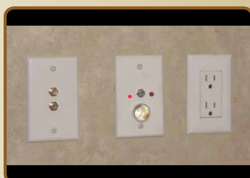
Interior Audio Hook-Up for TV to Speakers, Pre-Wired for Cable and TV Antenna Booster
